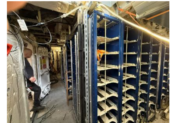
New Echandia battery system install
